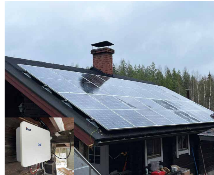
8kW Solar System in Finland (XG8KTR)
